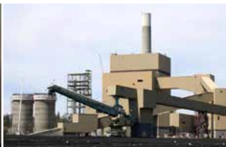
Atikokan GS biomass conveyor and storage silos
