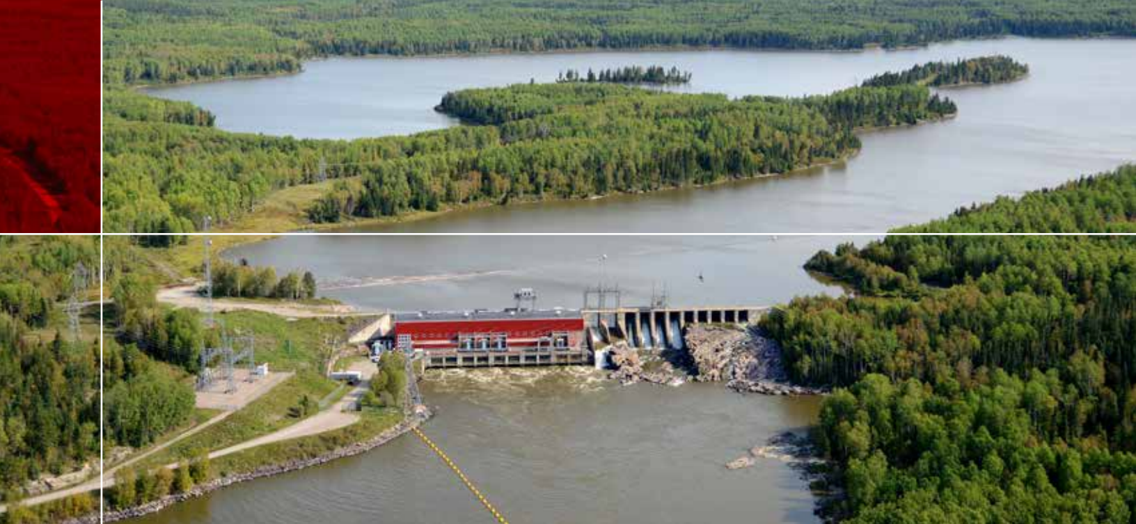
Manitou Falls Generating Station
