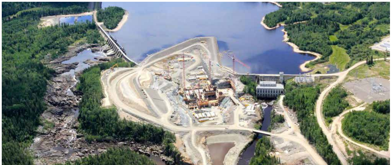
Smoky Falls new generation construction.
